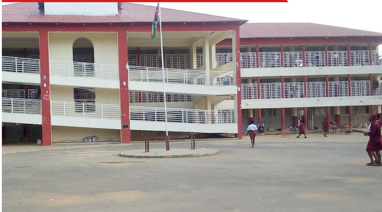
■ A classroom block in a Girls' National School, Western Region.
